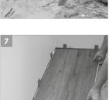
INSTALL THE LAST PIECES OF ROWS 1 AND 2 Cut to fit, maintaining the expansion gap. Install as before. Move the entire assembly against the spacers on the starting wall.
