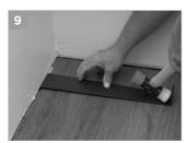
INSTALL THE LAST ROW Cut the final row of planks to fit along the wall. Use a pull bar to lock the long edges together. Do not use the pull bar on the short edges.
