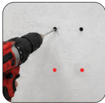
Drill 4 holes to a depth of under 60mm
