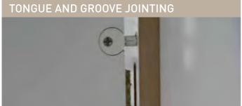
All the solid b ks nd b ses re assembled ith tongue a d groove joint with multiple cam fix points. This creates exceptional strength and durability particularly for wall mounted cabinets. The tongue and groove joint prevents the side from pulling away from the back when pressure is placed on the vanity top.
