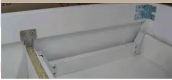
Specially designed internal brackets make a neat and strong finish which is much, much stronger than ugly staple blocks.
